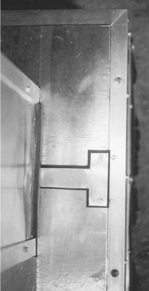
FIGURE 6-25. T-shaped gap cover for lower access panels.
